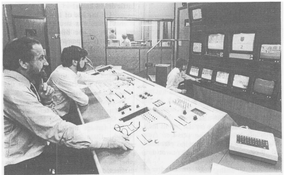
Tom Peckham and Mike Coy (centre) of SCPD seated at the control desk in TV Studio 1, while John Bloomfield, OUPC, adjusts the monitors. John was attached to SCPD for the installation.
