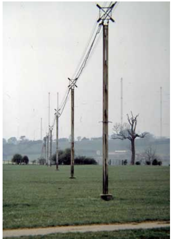
This photograph shows the Zo 220 Ohm overhead feeder from the T3 building on Borough Hill to the mast at Dodford, some 2.13 km (7000 feet) away. There was a loss at 647 kHz of 15 kW on this run!
