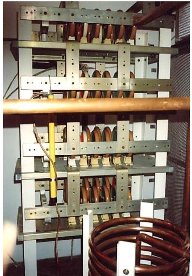
**Figure 4. Physical realisation of a rejector.**
