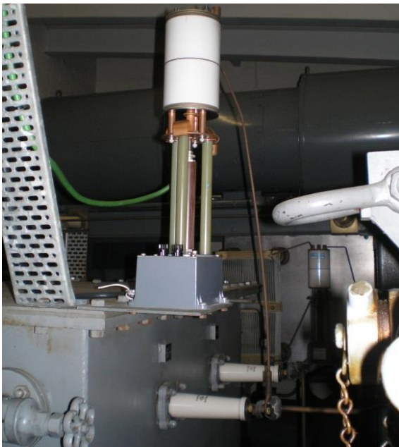
Figure 3. An 'un-illustrated' crowbar switch in the MWT BD272 sender
